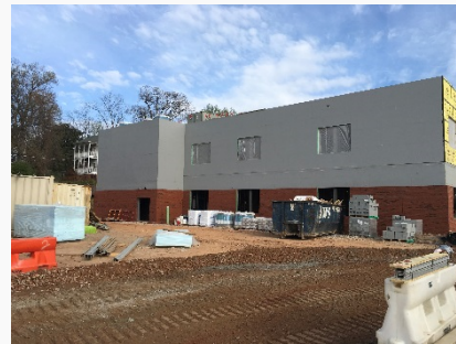
Exterior Framing, Sheathing, Air Barrier, & Brick
