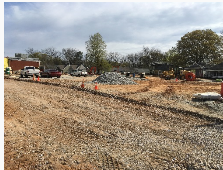
Preparing Parking Lot and Drive for Binder and Asphalt
