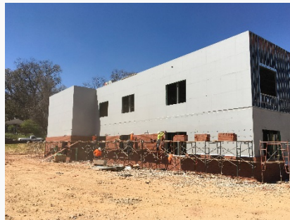
Exterior Framing, Sheathing, Air Barrier, & Brick
